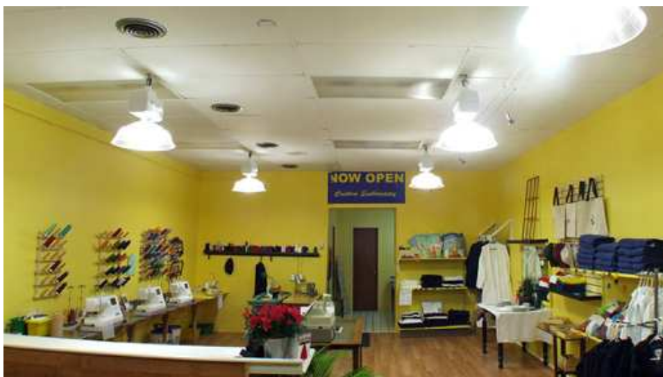
INDUCTION LIGHTING LOW-BAY FIXTURES IN USE IN A RETAIL STORE WHERE THEY REPLACED 4-TUBE FLUORESCENT “TROFER” TYPE LIGHTS. IN THIS APPLICATION, THE STORE REDUCED ENERGY COSTS BY 37% WHILE INCREASING LIGHT LEVELS BY 55%.
